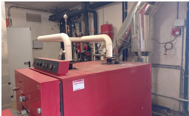
Figura 2: Calderes de gasoil existents.
