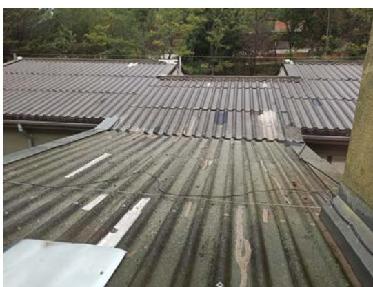
Img.5 i 6 – Coberta fibrociment i faldons verticals
