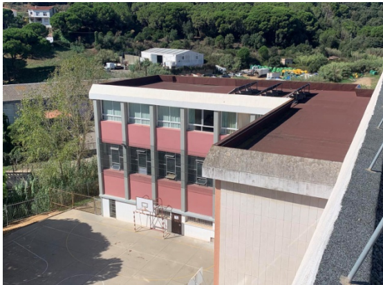
Coberta bloc occidentals, interior
