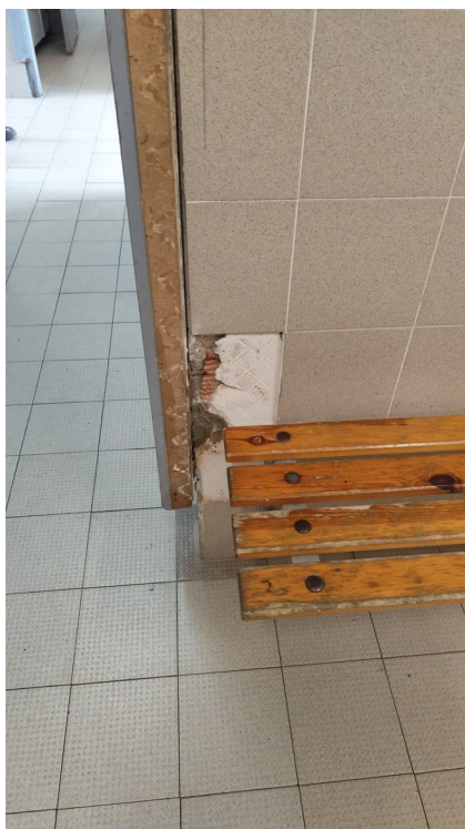
Reparacions a executar
