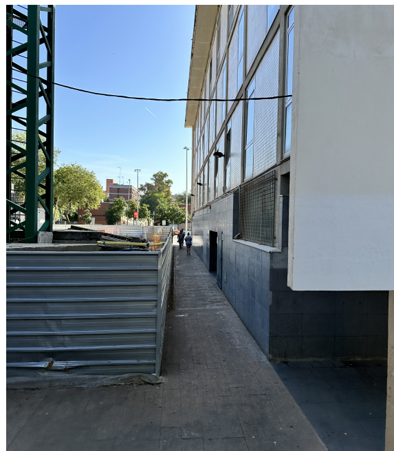
Cala: tancament exterior
