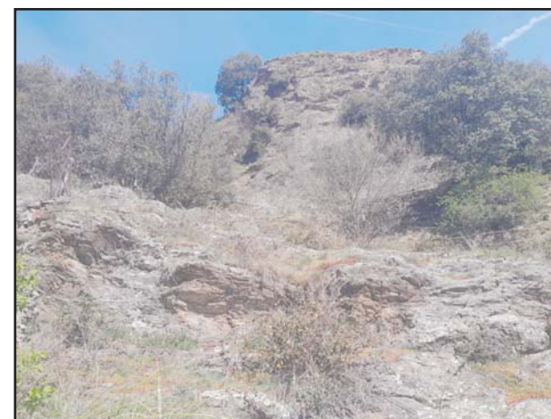
Figura 2. Vista general aflorament.
