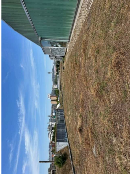
10 Vista general coberta
