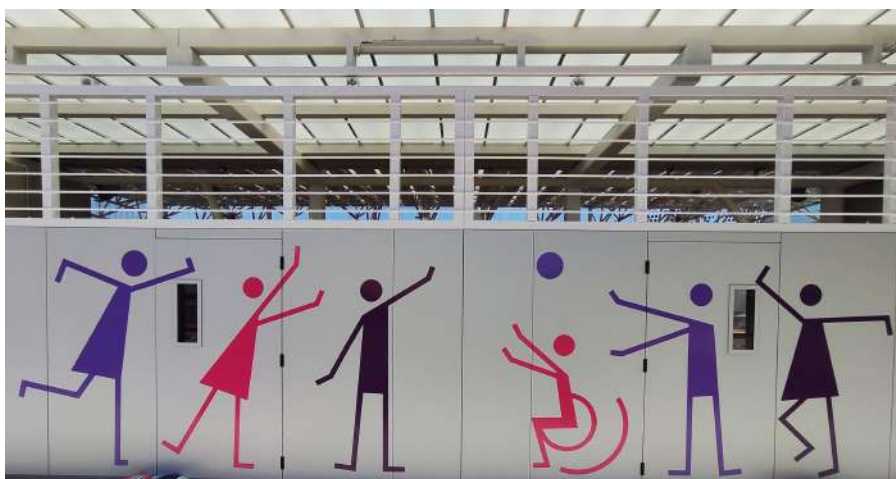
Vista interior portes corredisses sud
