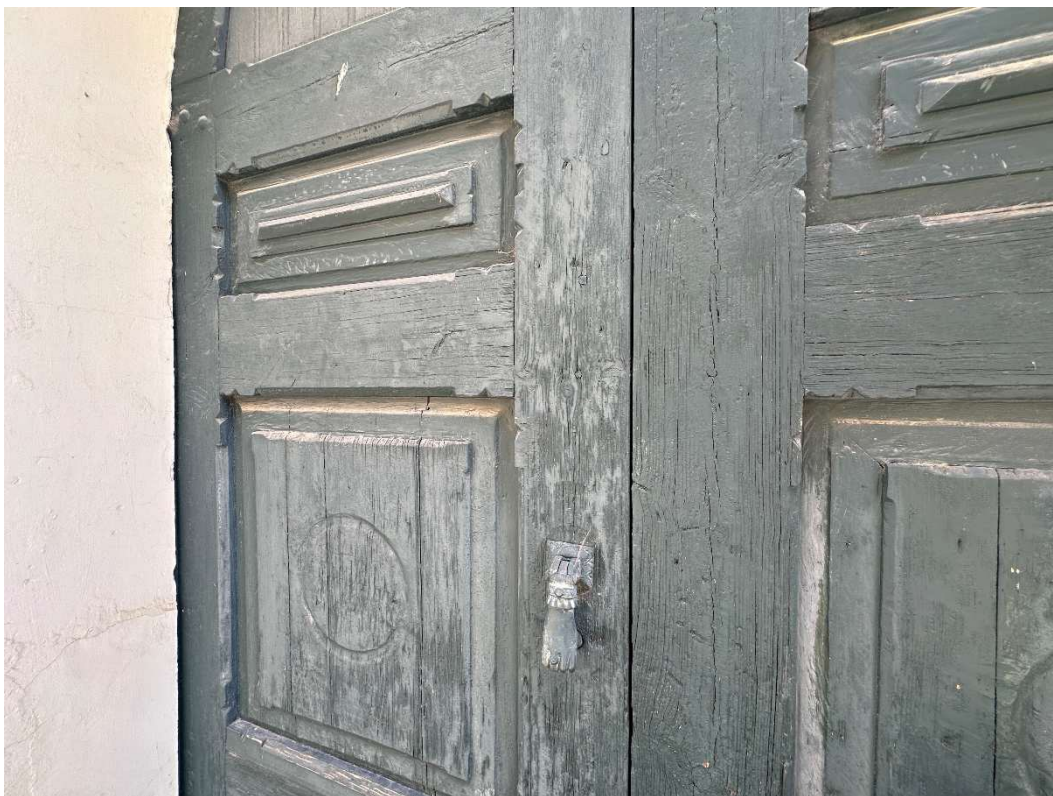
Detall porta façana principal
