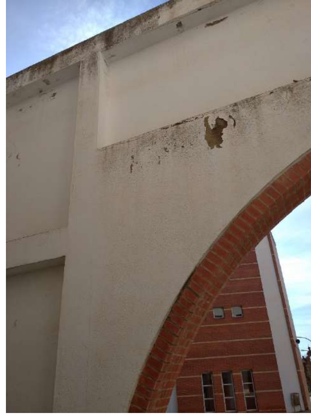
Pati interior, mur central
