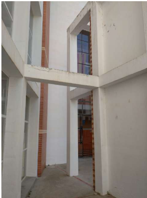
Pati interior, mur central
