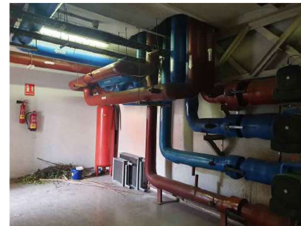
BOMBES PRIMARI, CIRCUIT PRIMARI I MUNTANTS
