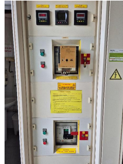
Detall portes quadre general BT
