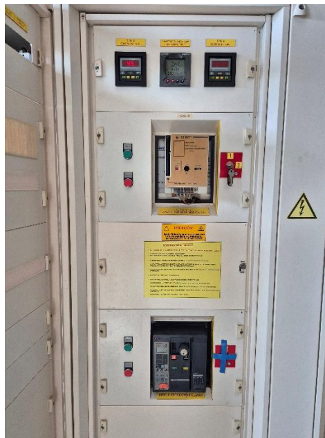
Detall portes quadre general BT
