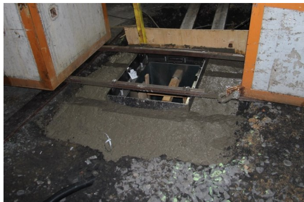
Picture 10: Casting of concrete
