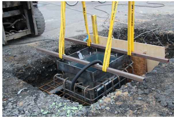
Picture 9: Insertion of metal housing into foundation pit
