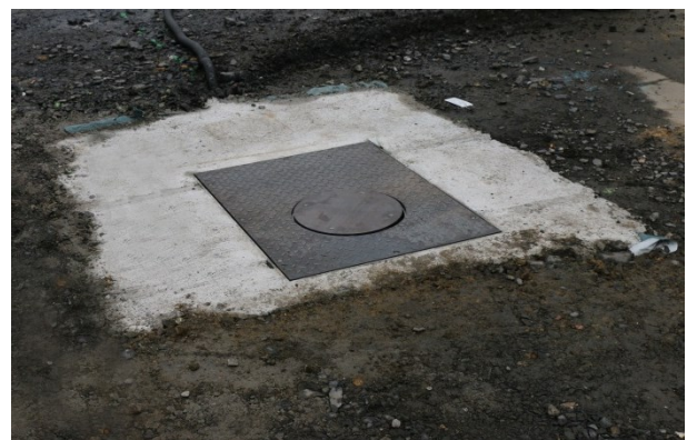
Picture 18: Bollard with installed cover plate
