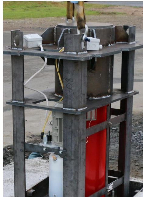
Picture 5: Lifting with shackle and sling
