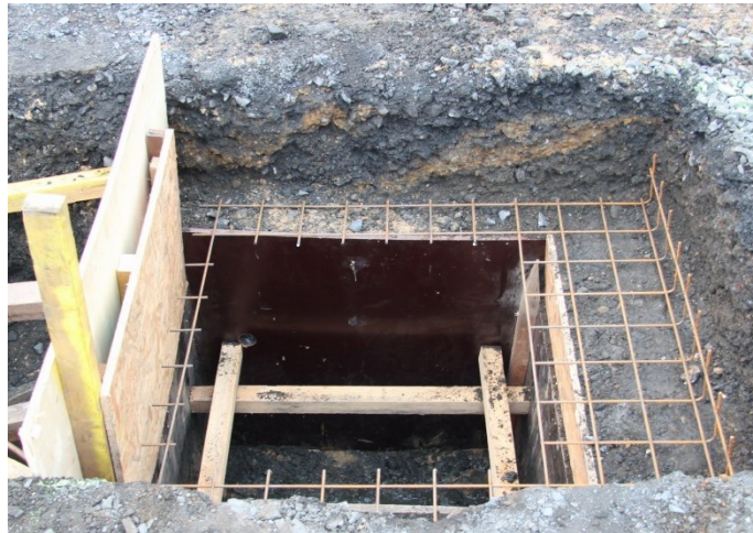
Picture 7: Foundation pit with bottom reinforcement layer
