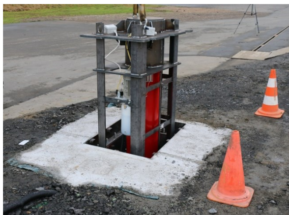
Picture 11: Insertion of bollard assembly
