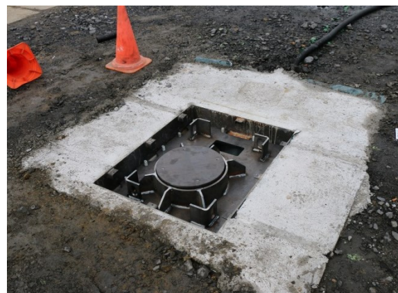
Picture 12: Installed bollard assembly
