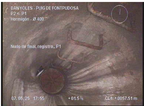
P2-P1_0989083b-aa3c-403b-93a4-45a75ccf156e_20250507_180501_706.jpg, 00:05:23, 57.50m Nudo de final, registro,, P1
