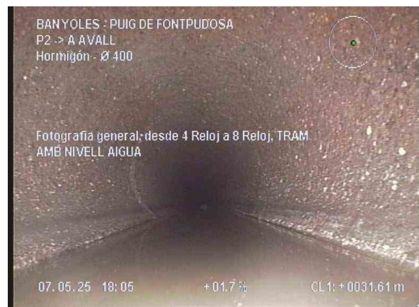
P2-A AVALL_feb603a0-e1ac-41cc-883a-70681775b64c_20250507_181524_683.jpg, 00:03:37, 31.60m
