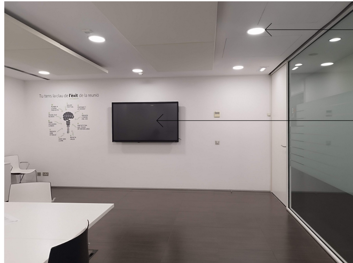
Focus tipus downlight encastrats
