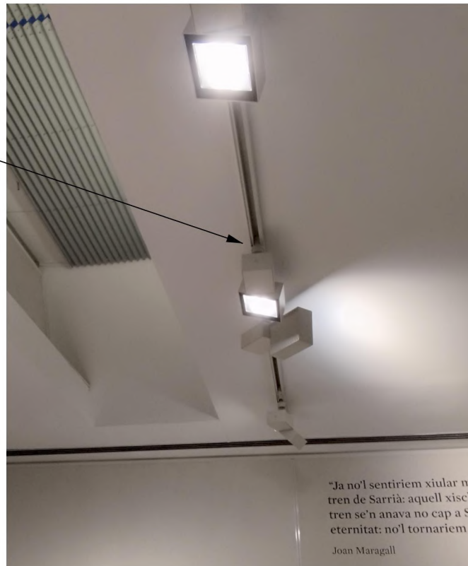
Reaprofitaments carrils i focus existents - Erco
