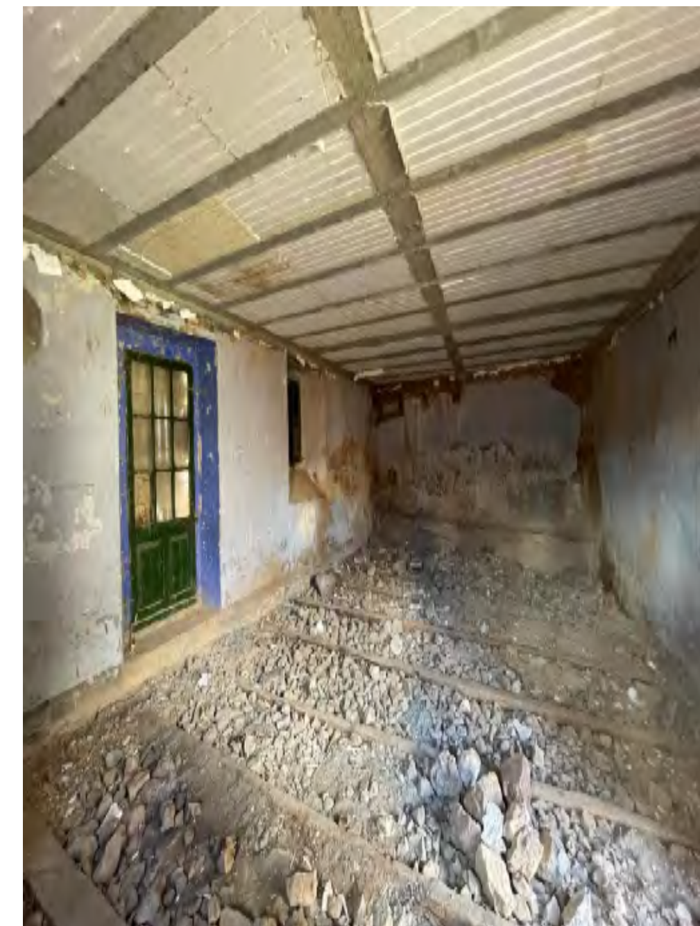
Interior local, al fons paret contraterrer
