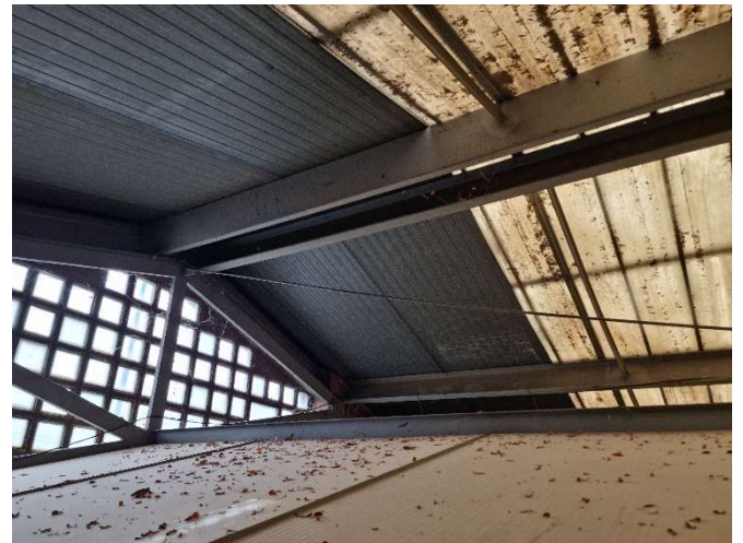
Vista interior coberta
