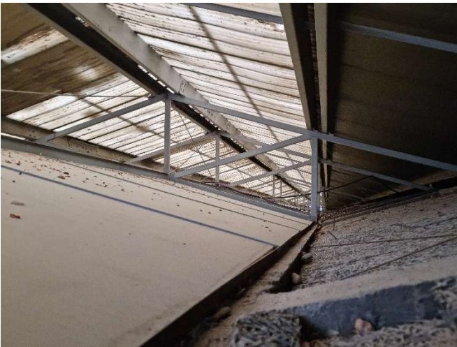
Vista interior coberta
