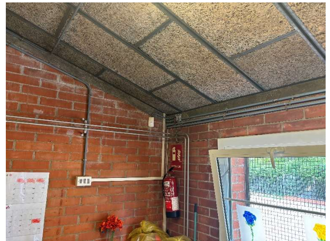
Detall interior coberta
