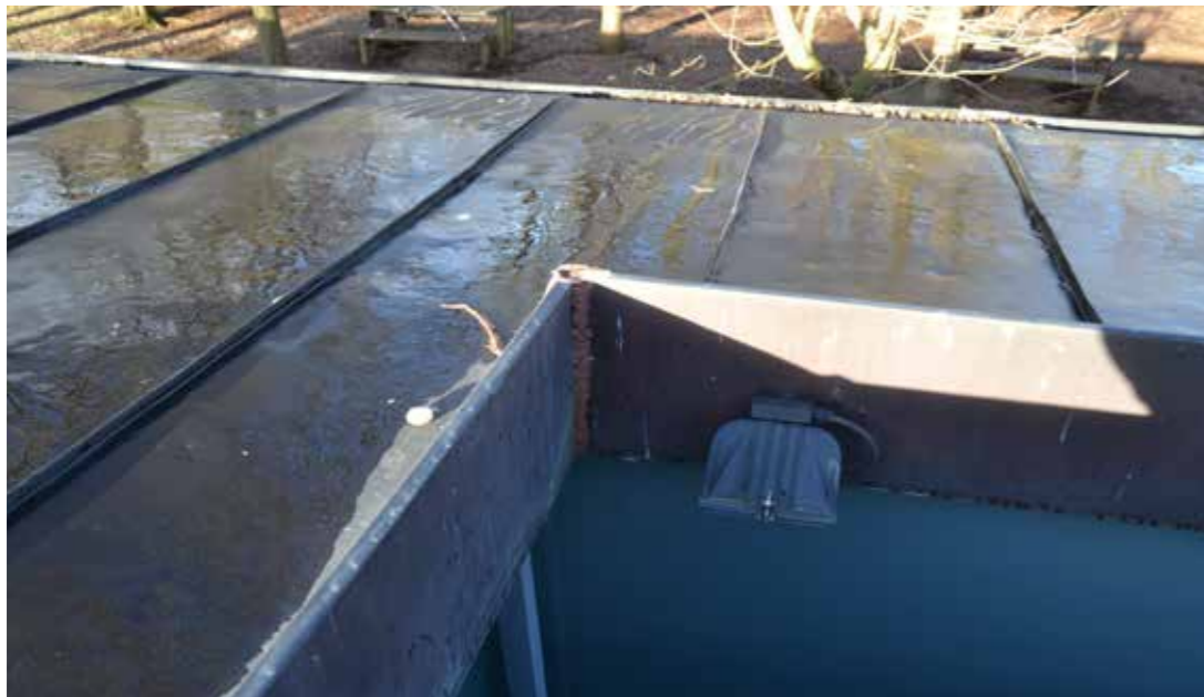
CANTONADA INTERIOR PATI
