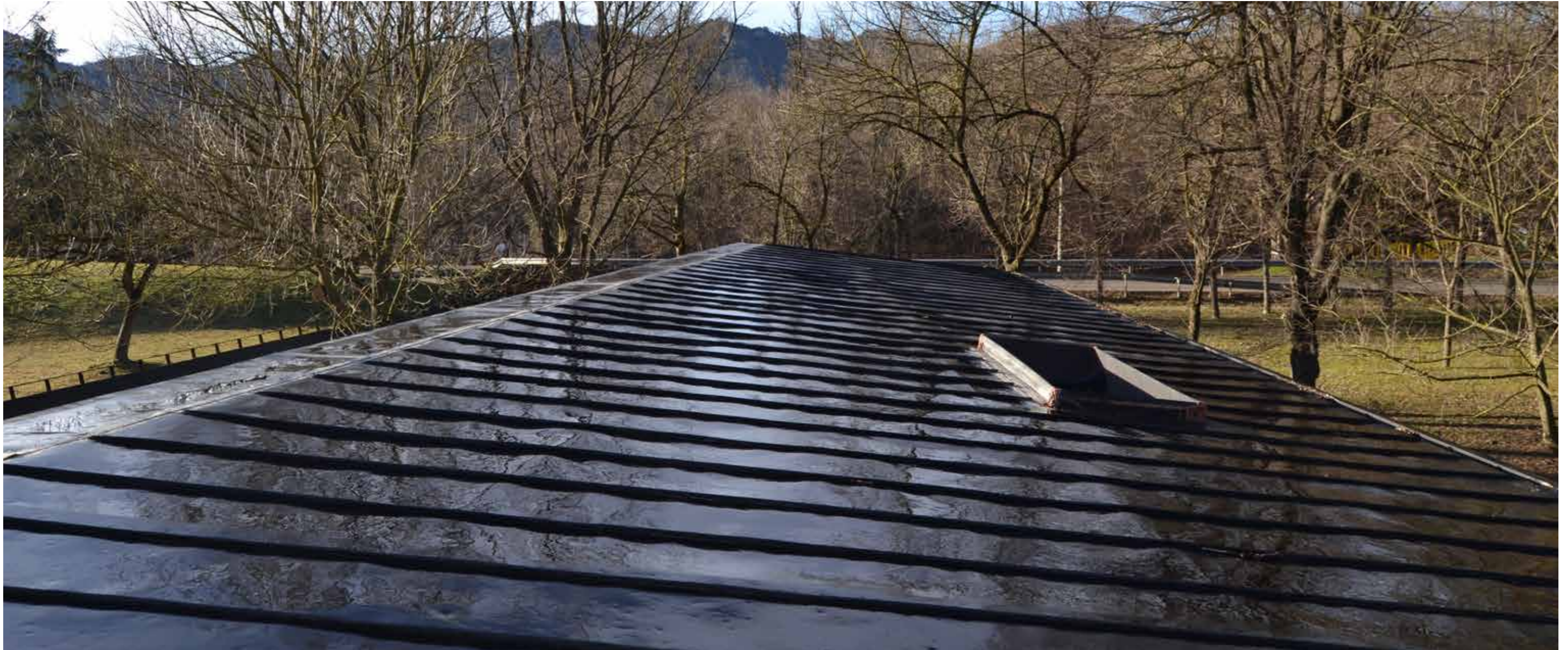
VISTA GENERAL COBERTA
