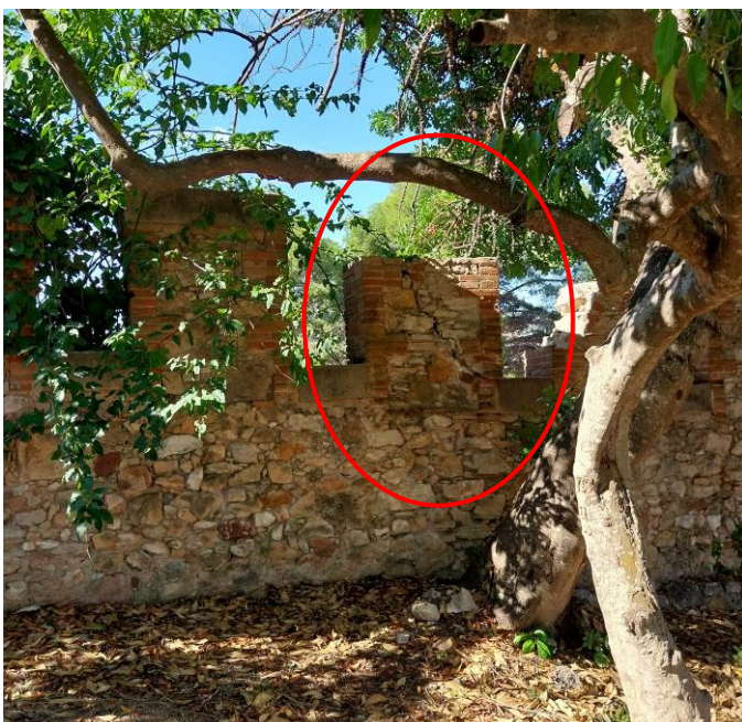
Vista exterior muralla
