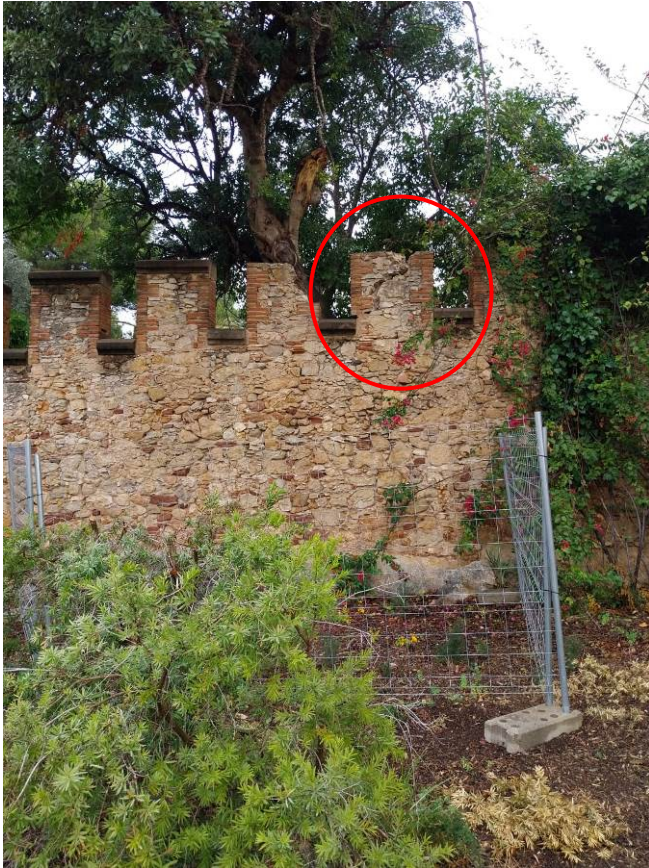
Vista exterior muralla
