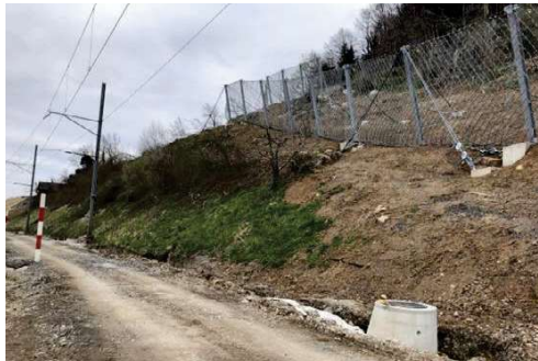
Barrier, seen from below (Image: [H]).
