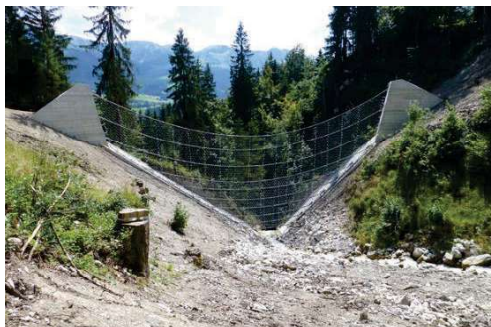
Barrier, upstream side (Image: [F]).
