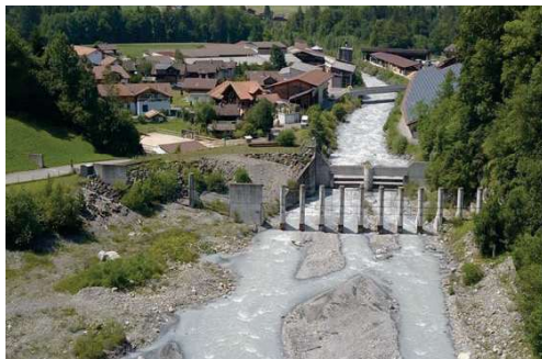
Barrier, upstream side (Image: [F]).
