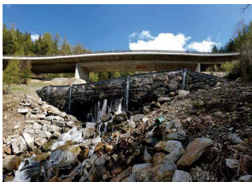
Pre-filled UX-180-H6 barrier, seen from downstream (Image: [G]).
