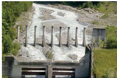
Barrier, downstream side (Image: [F]).
