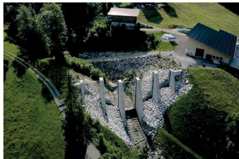
Barrier, downstream side (Image: [F]).
