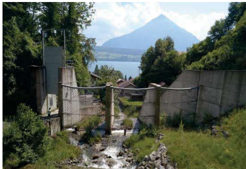
Barrier, upstream side (Image: [F]).
