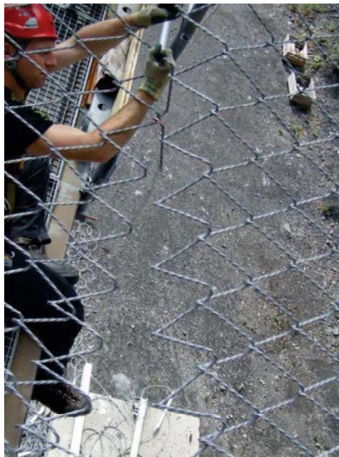
A separation is produced in the net area
