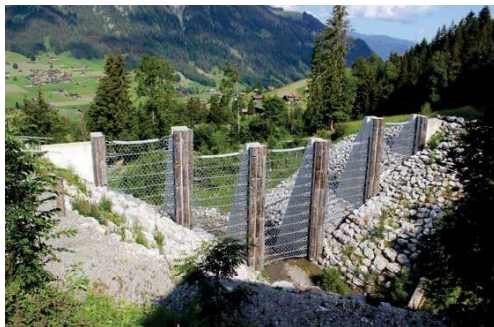
Barrier, upstream side (Image: [F]).
