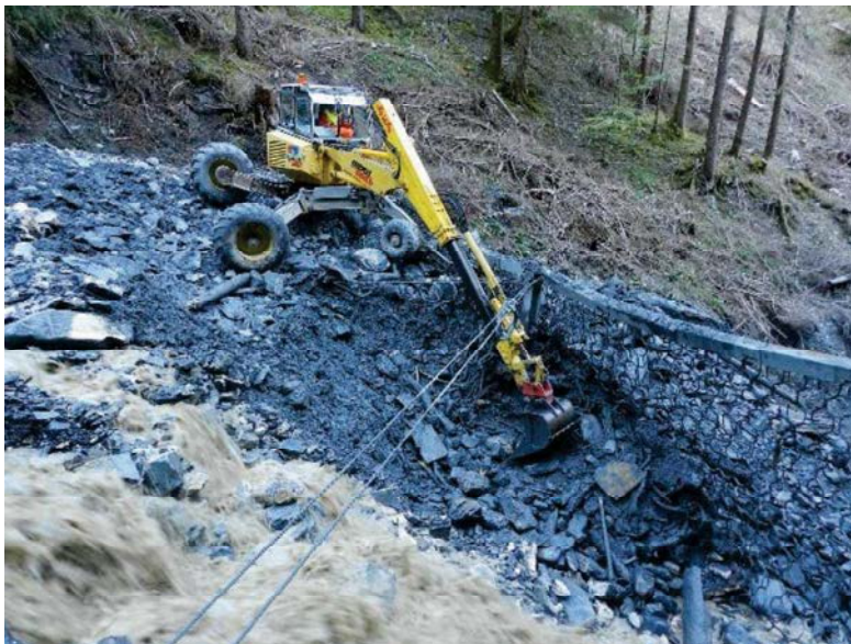
Emptying a debris flow protection net from the uphill side with a walking excavator
