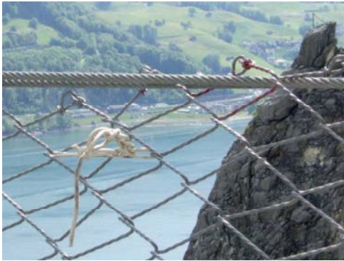
a) Relieve the strain on the outermost spiral of the damaged area
