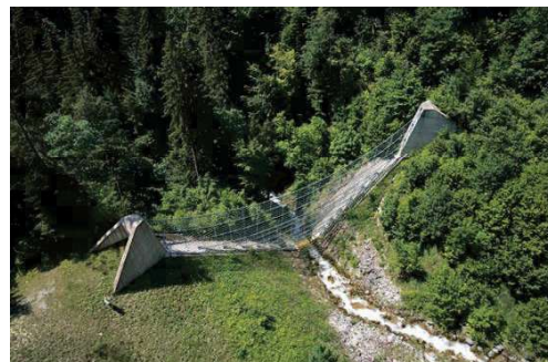
Barrier, downstream side (Image: [F]).
