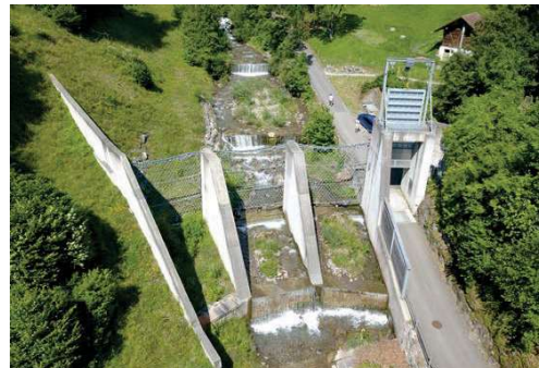
Barrier, downstream side (Image: [F]).
