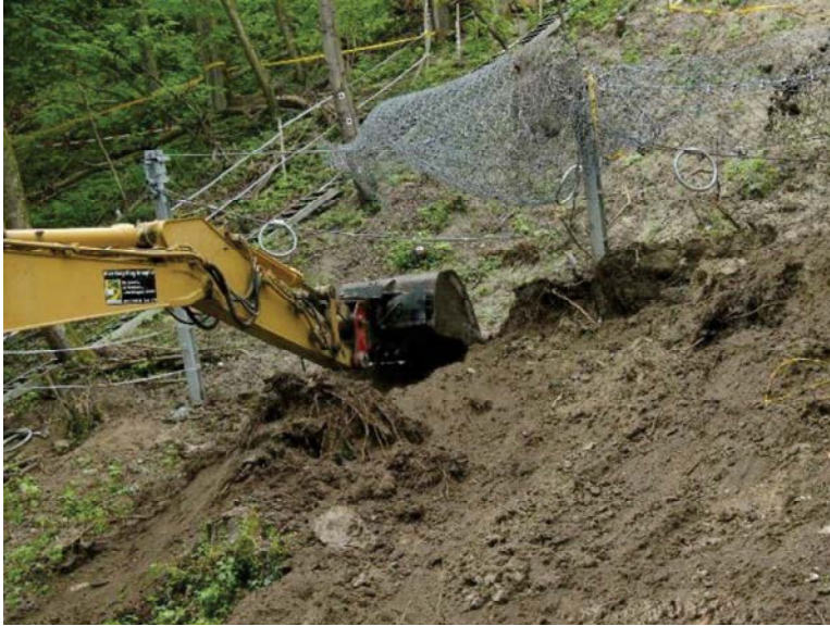
Emptying a shallow landslide protection net from the valley side with an excavator
