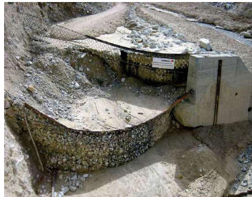
Restoration of the wing on the flanking wall and installation of a second, partially filled VX barrier (Image: [A]).
