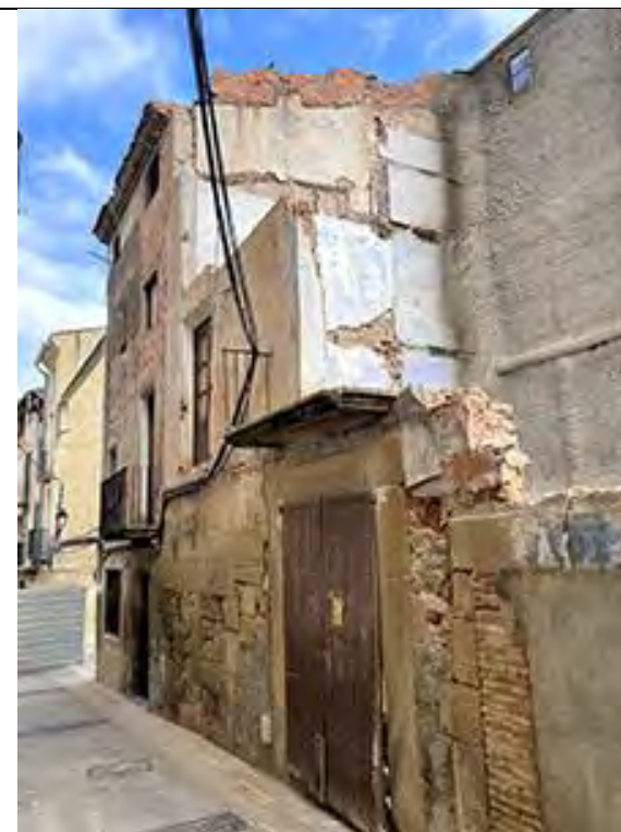
Vista del Carrer Major, 2
