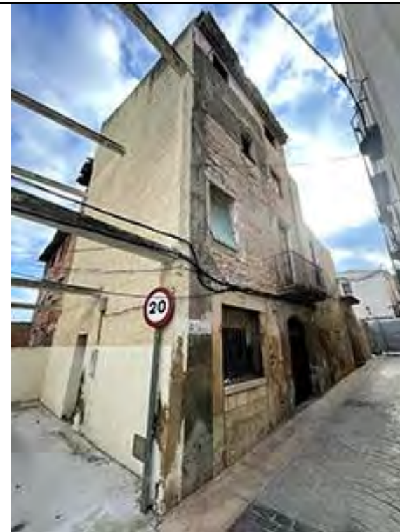
Vista del Carrer Major, 4
