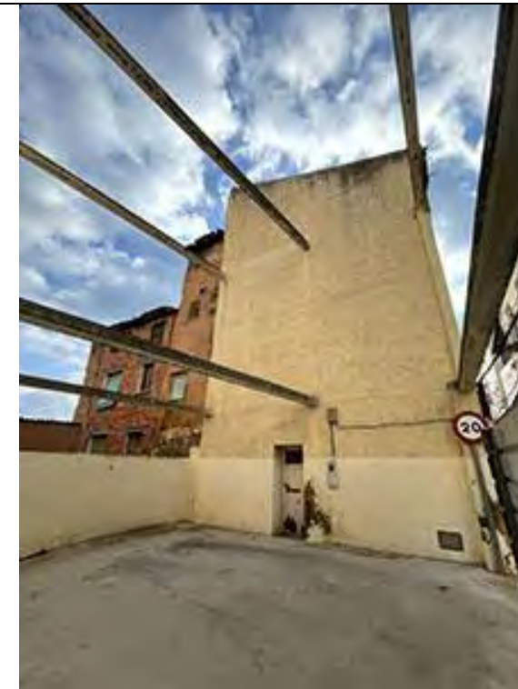
Vista del Carrer Major, 4 des del solar lateral
