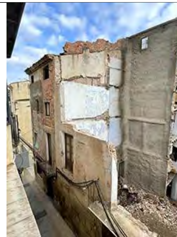
Vista interior del Carrer Major, 2
