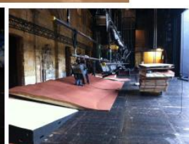
multiplex panels zone with sculpted polystyrene coated and covered with painted cork.
