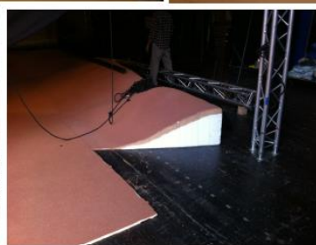
multiplex panels zone with sculpted polystyrene coated and covered with painted cork.
