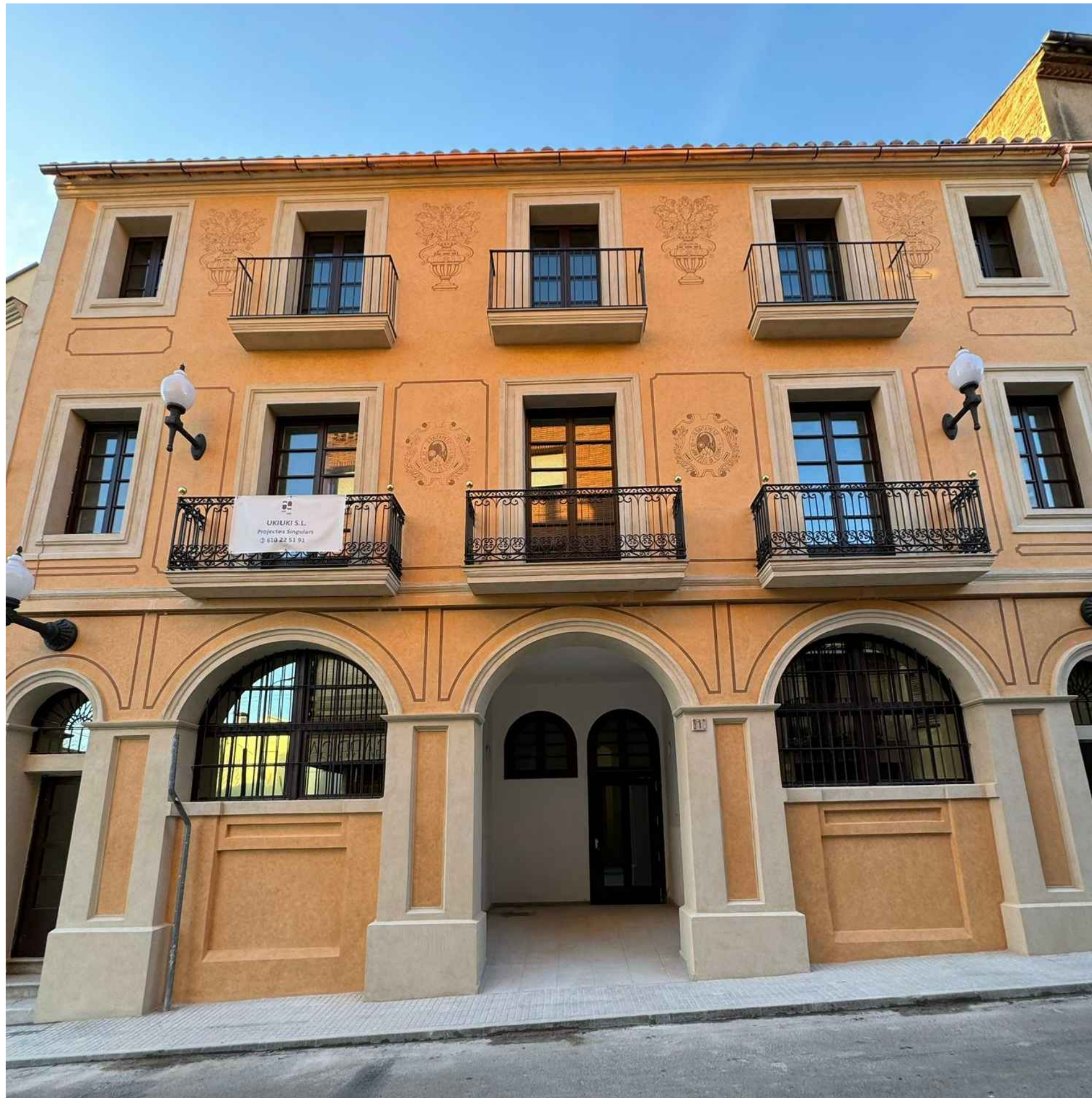
Façana principal C/Vic, 1
