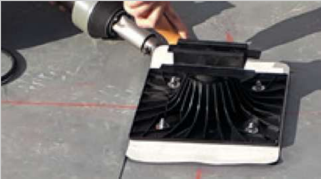
2. Weld the other side of the base panel over a minimum width of 3 cm
