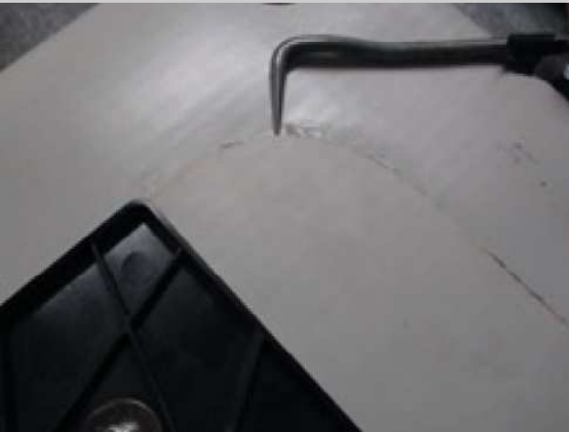
3. Verify the quality of the welds using the tester after cooling
