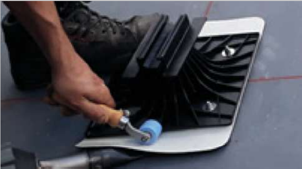
1. Weld one side of the base panel over a minimum width of 3 cm
