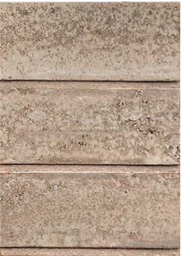
Junta rehundida Raked joint
