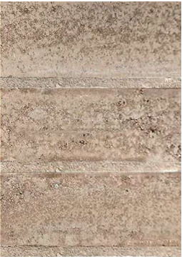
Junta enrasada Flushed joint
