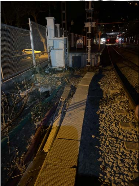
PRISMA FORMIGONAT FORMANT PASSER (80m)
