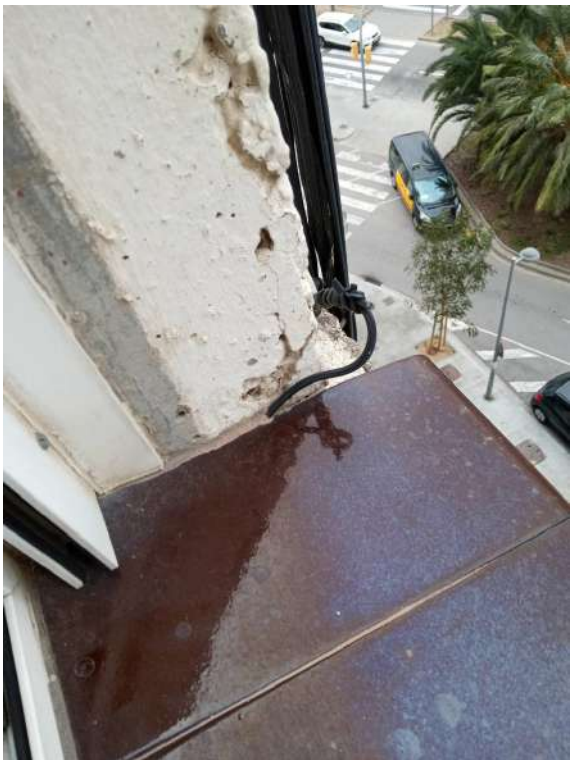
Tancament façanes panell
