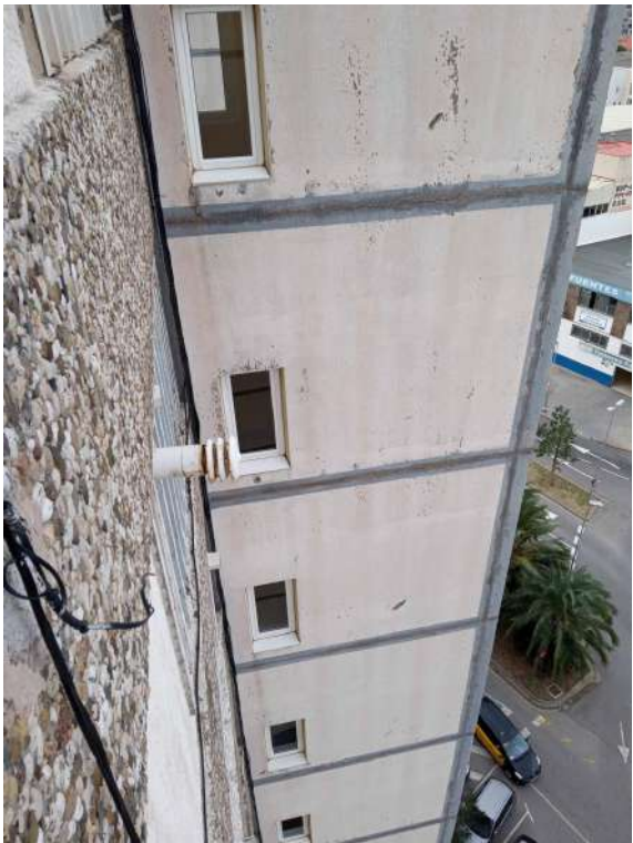
Vista general portes 2a
