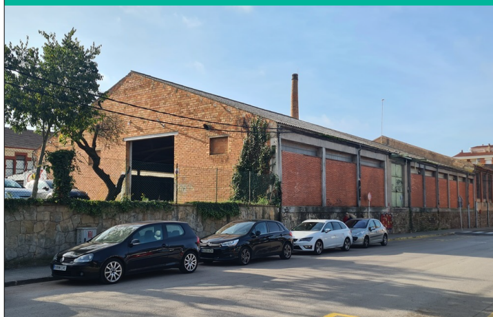
NAU INDUSTRIAL "CAL SITGES"
