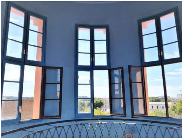
Finestres practicables. Vista interior
