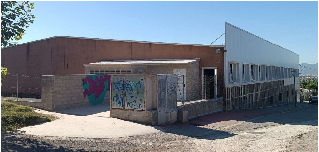
Fig. 22 Vista general armari CGP i TMF existent
