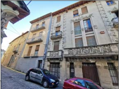
VISTA GENERAL FAÇANA PRINCIPAL
