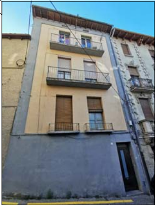
VISTA FAÇANA PRINCIPAL N°16
