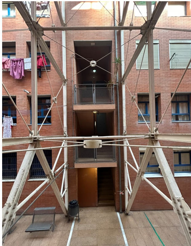
F2 – Façana a pati interior
