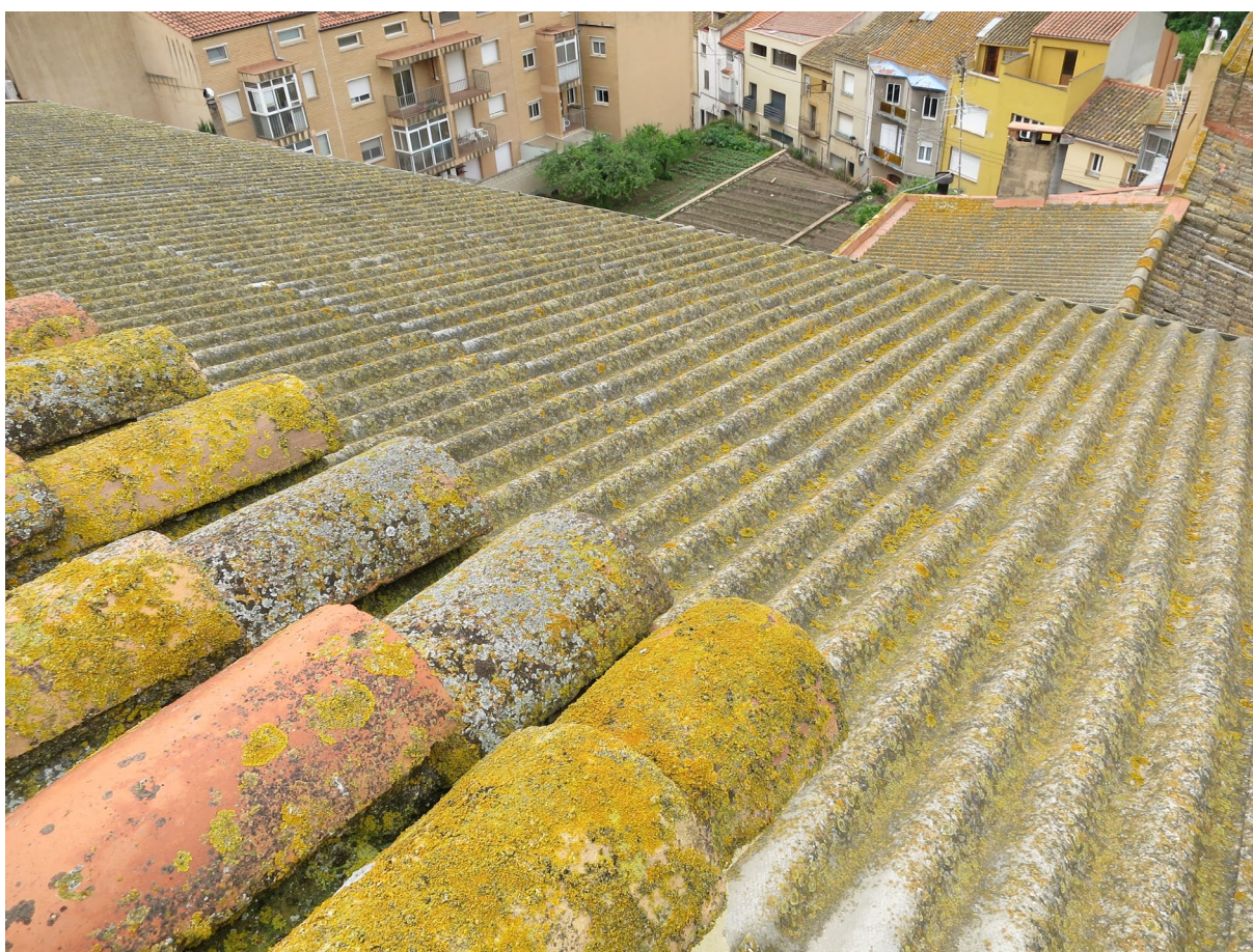
Coberta de fibrociment
