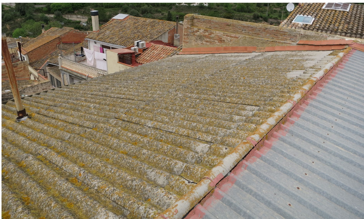
Coberta de fibrociment
