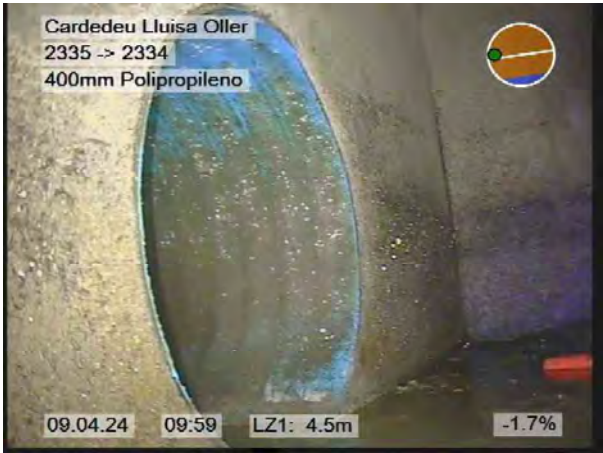
25.jpg, 00:00:53, 4.50m POZO FINAL SIN ACOMETIDAS
