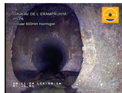
P5 A P6_1afec735-c005-4f00-b614-991d65ae4fbd_20241129_084542_459.jpg, 00:06:22, 50.10m Nudo de final, registro., P6
