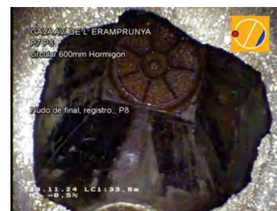
P7 A P8_8c5f08ad-715d-49c6-af49-8fa772f50931_20241129_090337_261.jpg, 00:04:43, 33.80m Nudo de final, registro., P8
