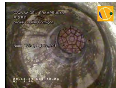
P10 A P11_ea1f0c9f-29a0-4df6-84a7-88acc49dae1d_20241129_10206_965.jpg, 00:05:07, 43.20m Nudo de final, registro., P11
