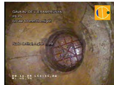
P8 A P9_fa8dc154-0f95-487d-8044-929b56d3abf6_20241129_090 651_675.jpg, 00:01:39, 11.20m Nudo de final, registro., P9
