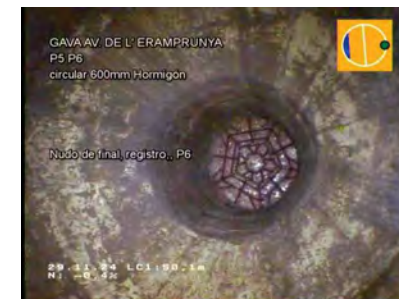
P5 A P6_11ac728d-4ba1-4789-9790-f699cbef28dc_20241129_084528_120.jpg, 00:06:22, 50.10m Nudo de final, registro., P6
