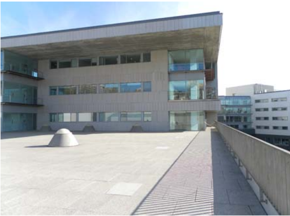
13. Vista Pati Hospital Nou
