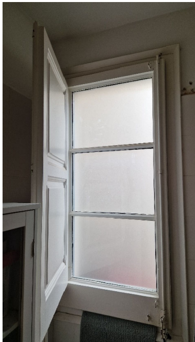
5-1 Vista interior finestra bany
