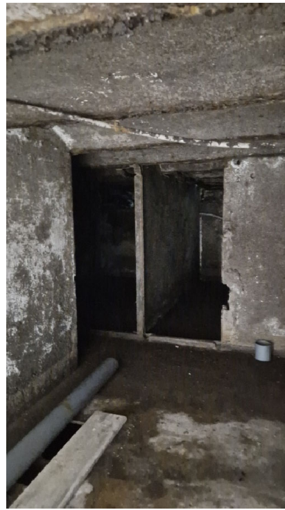
Vista general superior i envans a enderrocar.
