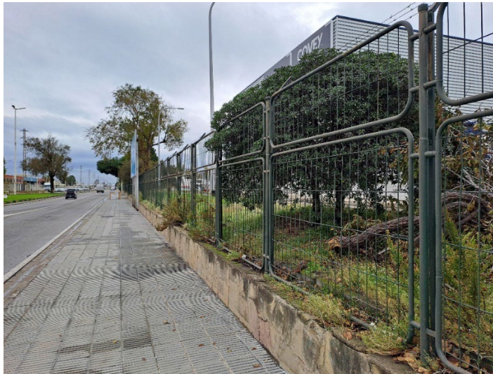
Tancament existent vista general
