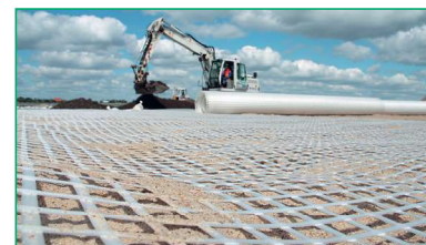
Figure 13 Secugrid® installation
