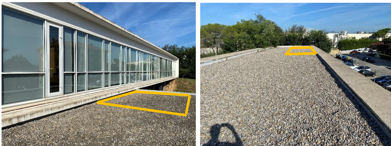
Abassegament de material a coberta 1 i 2
