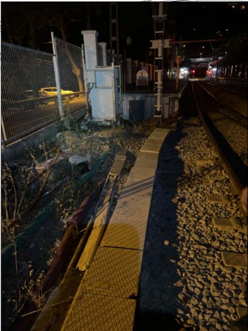
PRISMA FORMIGONAT FORMANT PASSER (80m)
