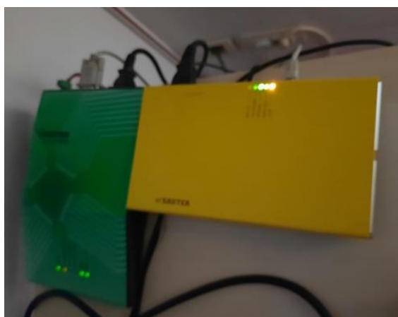
Controladors bus 3600 a Bacnet
