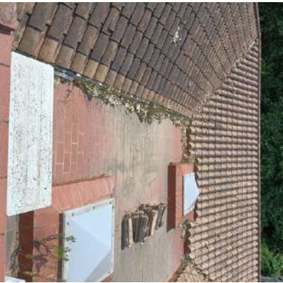
Vista general coberta
