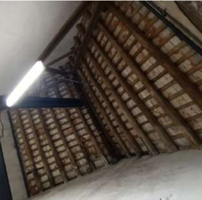
Acabat interior coberta
