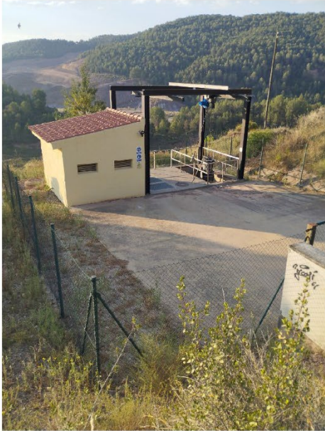
Vista general de EBAR
