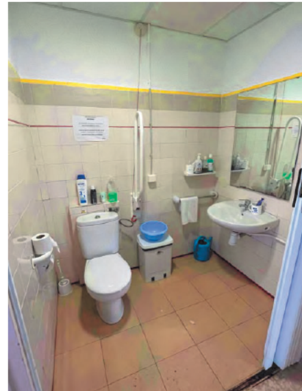
Bany a rehabilitar
