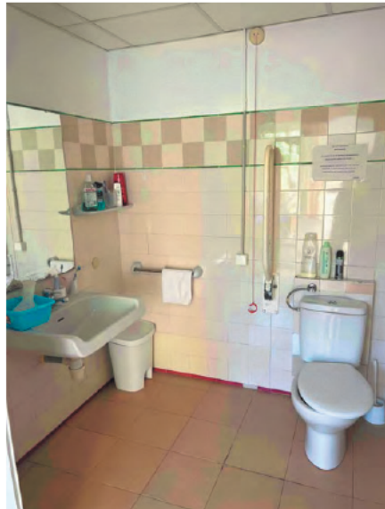
Bany a rehabilitar
