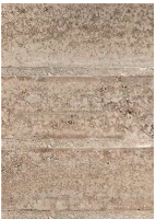
Junta enrasada Flushed joint
