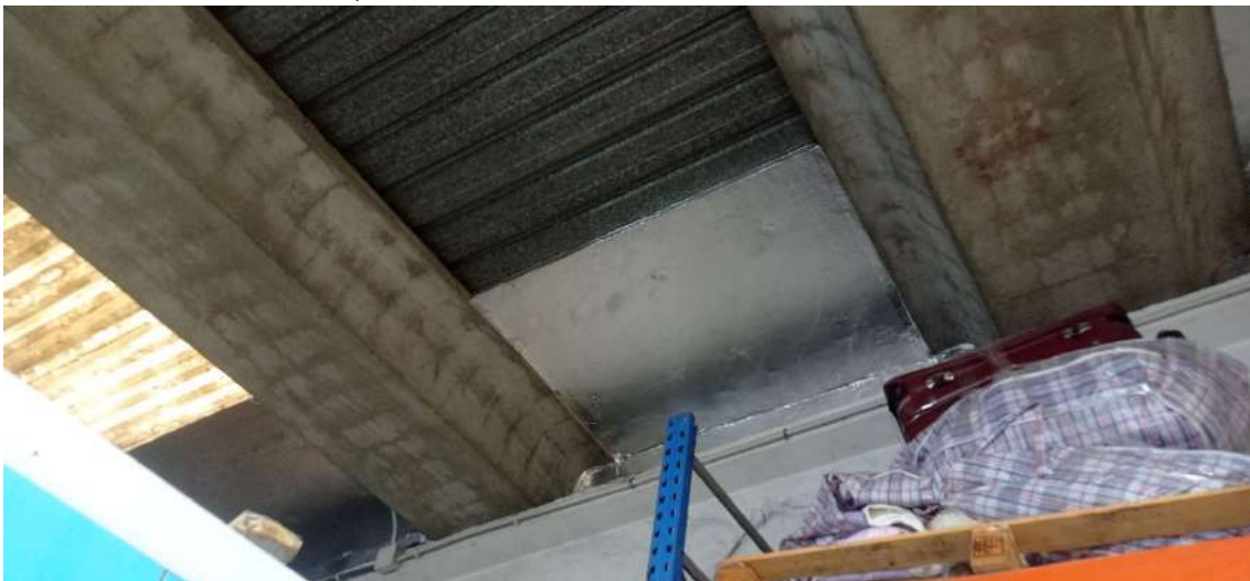
INTERIOR SOSTRE- BARRERA IGNIFUGA
