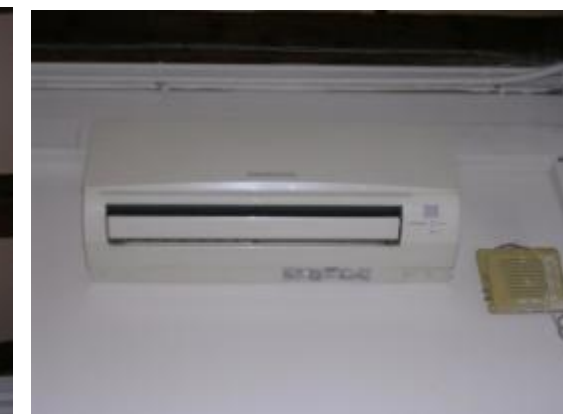
006 Sala Piano costat sala Felip Pedrell p3 Gardunya
