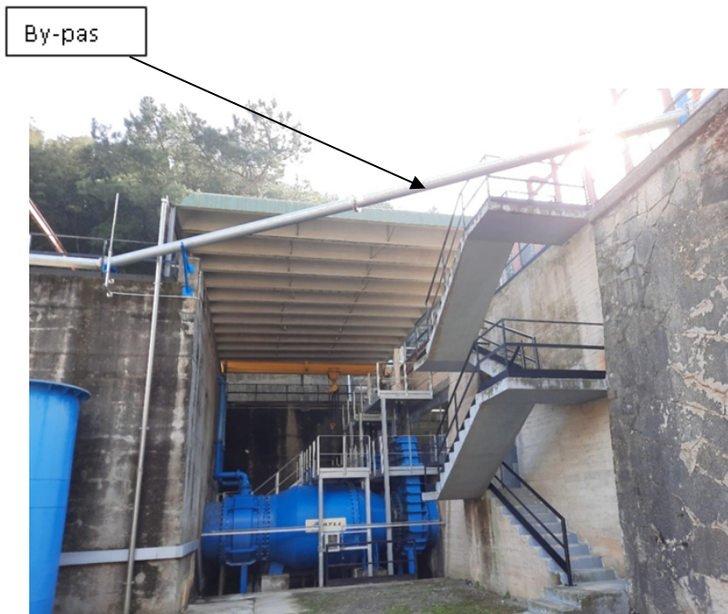
CANONADA AÈRIA DN 200mm BY PASS A DESMUNTAR
